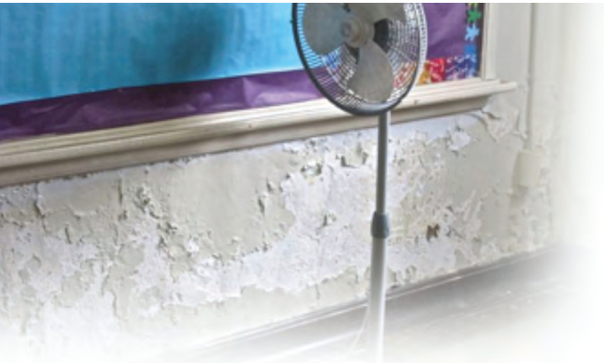
Southeastern PA elementary school with peeling lead paint (J Roseman, AFT consultant)
